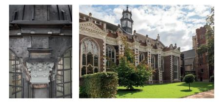
The Great Hall houses part of the internationally important library collection of the Church of England. The project undertook repair and conservation work to stone and brickwork and to the landmark two tier timber framed and lead covered lantern with its gilded weathervane. The interior has been transformed by a new marble floor with underfloor heating and by decorations. New lighting accentuates the magnificent hammerbeam roof.
